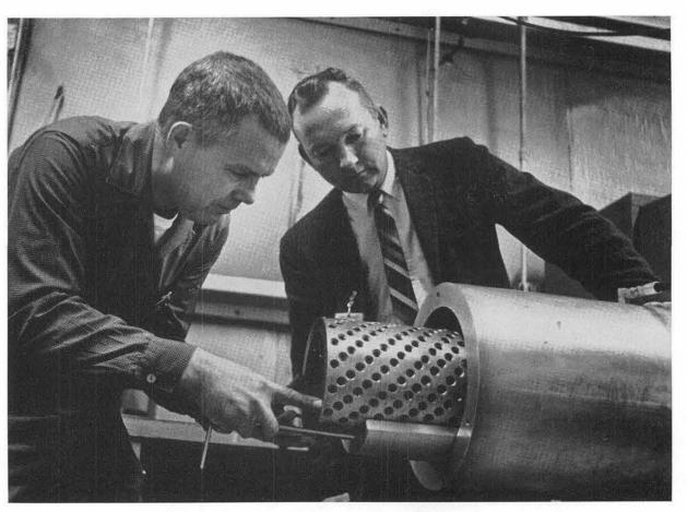
UNIQUE "metering sleeve," shown here being inserted into the breech of Sandia's 5.5-in, air gun facility, makes possible new kinds of shock testing with an air gun. Holes in the sleeve "program" the
